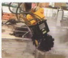
建筑物拆除 building demolition
