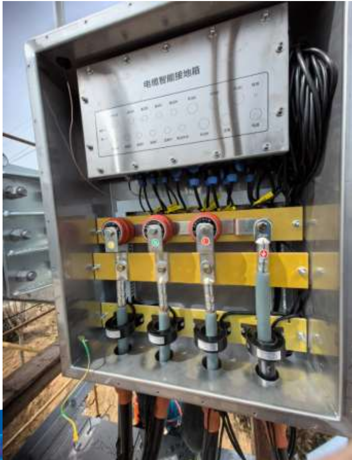
Intelligent Grounding Unit (IGUHV) for High Voltage Cables
