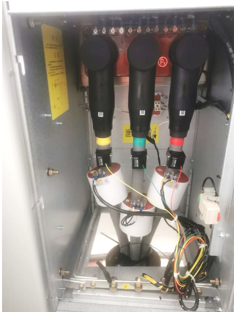
Installed temperature-sensing insulator plug
