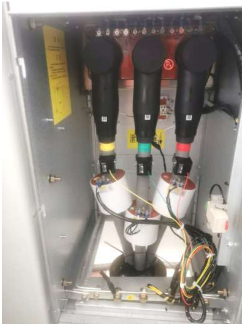
Installed temperature-sensing insulator plug
