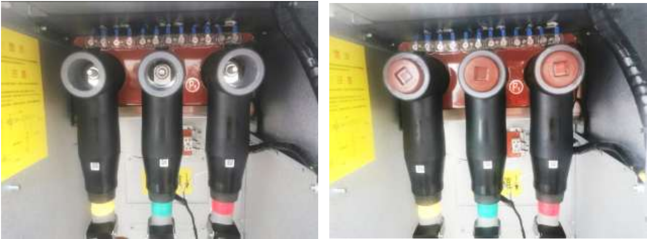
Before and after installing the temperature-sensing insulator plug
